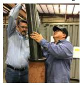
6. Ensure O-rings are installed in grooves on new cartridge. Grease the O-ring and threads with the appropriate anti-seize compound.
